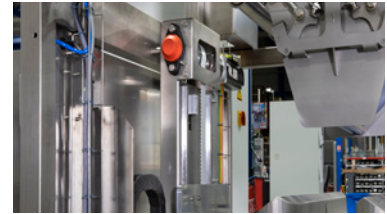
Box lift system to reduce drop distance
